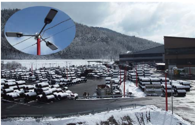
- for Outdoor Warehouses, Austria
